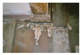
When dry rot is suspected a competent diagnosis of the situation can obviate unnecessary measures and provide appropriate recommendations for renovation work.
