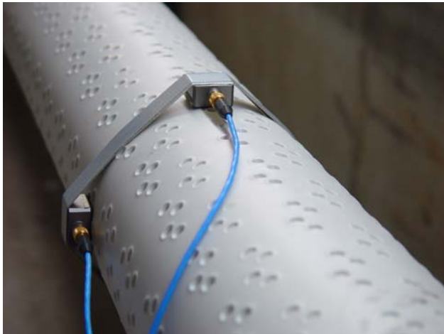
Measurement of vertical and horizontal cable vibrations using accelerometers.
