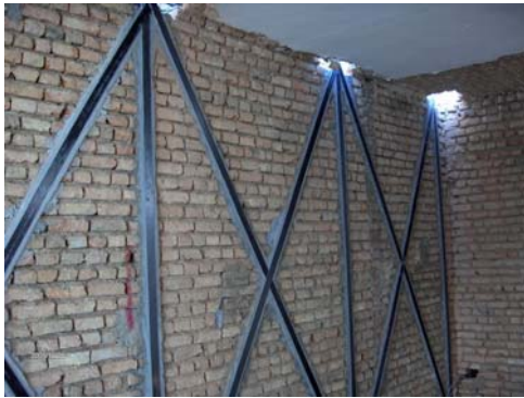
A building wall strengthened with carbon fiber reinforced polymer strips
