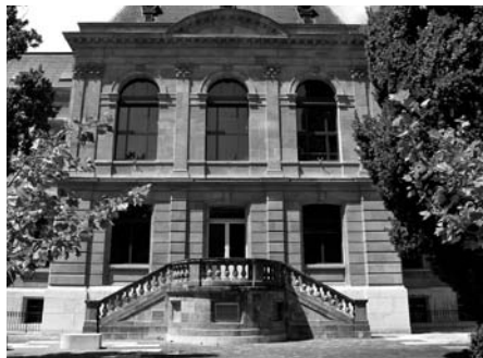
Figure 1: The main University building was energy retrofitted with special attention to its high architectural value.
