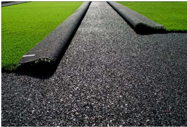
Laying of the artificial turf in Bürglen, Canton Thurgau.
