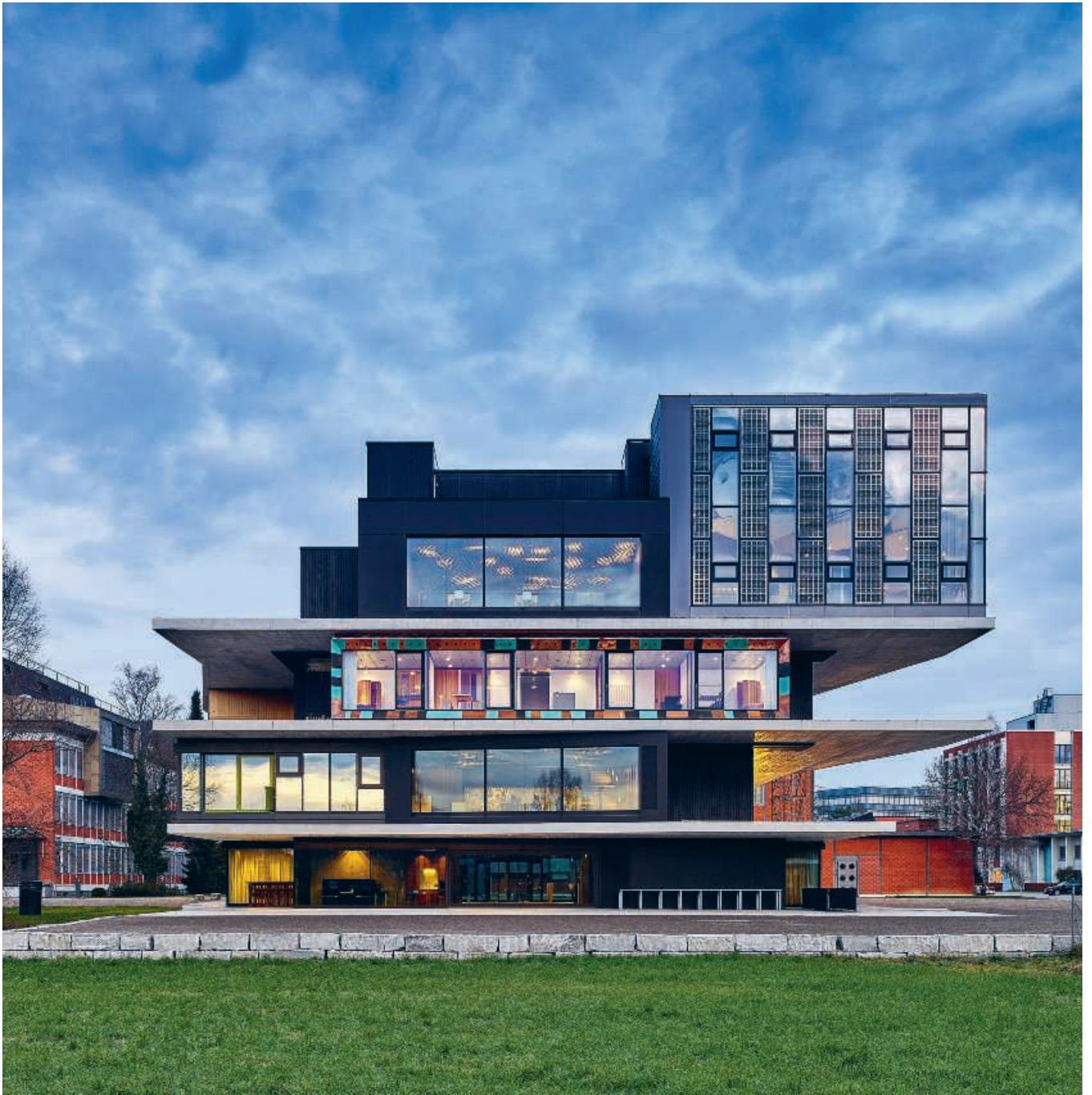
View of NEST from the east with the new units Solar Fitness & Wellness (3 rd floor on the right) and Urban Mining & Recycling (2 nd floor). Photo: Zoëy Braun, Stuttgart
