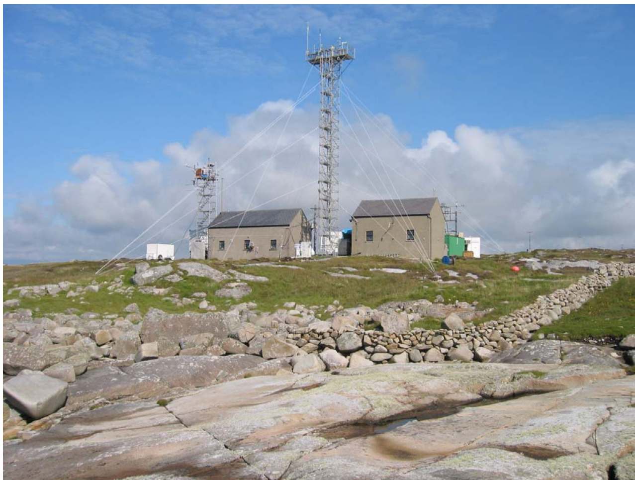
Figure 6: View of the main laboratory buildings at the Mace Head GAW station with the 10- and 23 m towers.
