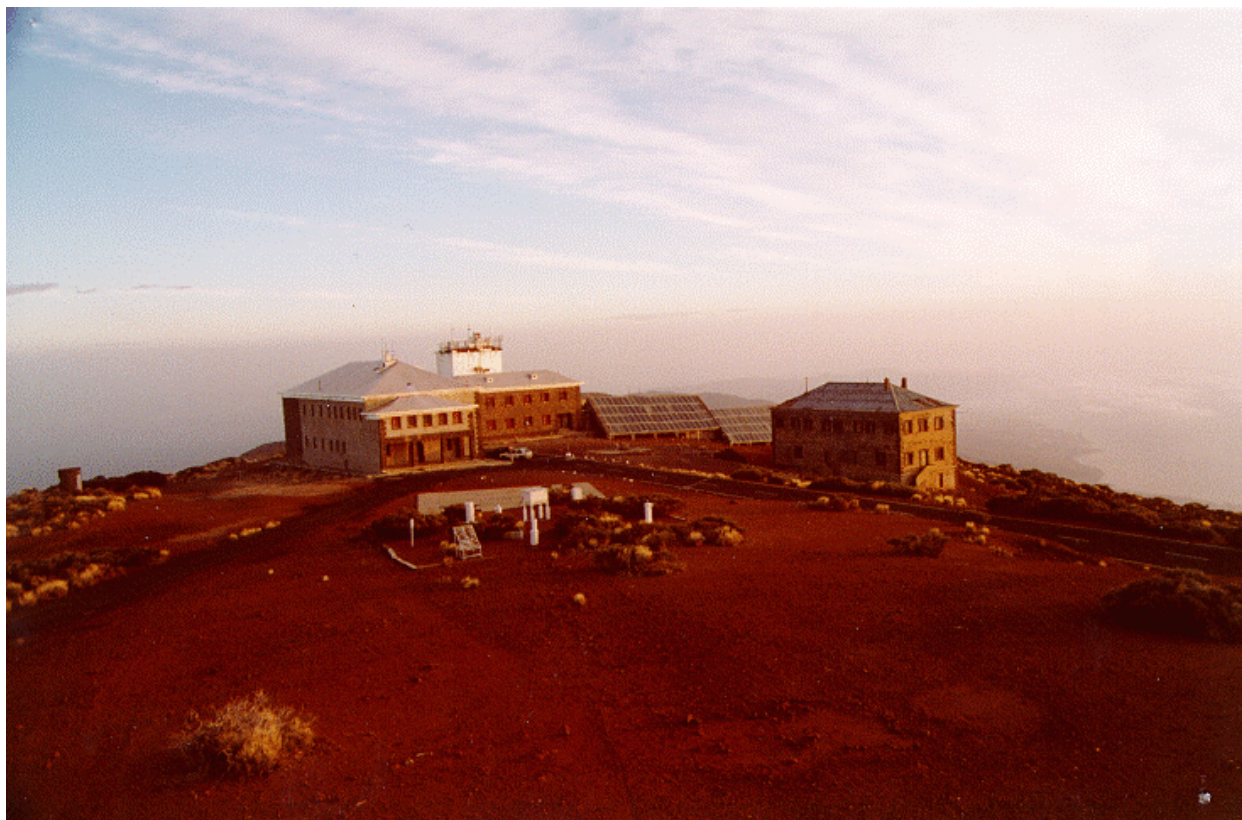
Figure 4: Picture of the station Izaña (view from the provisional station)
