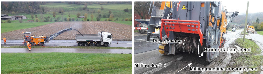
Fig. 69 Pavement milling (a) and key milling machine parameters (b)
