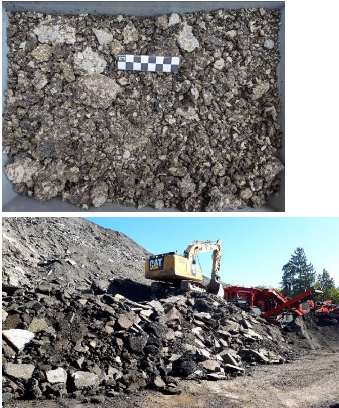
Fig. 51 An example of milled RAP (above) and slab/milled RAP blend (below)
