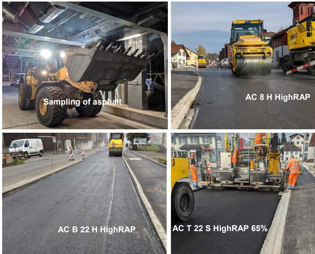
Fig. 107 Photos from the construction of HighRAP test section in Uster
