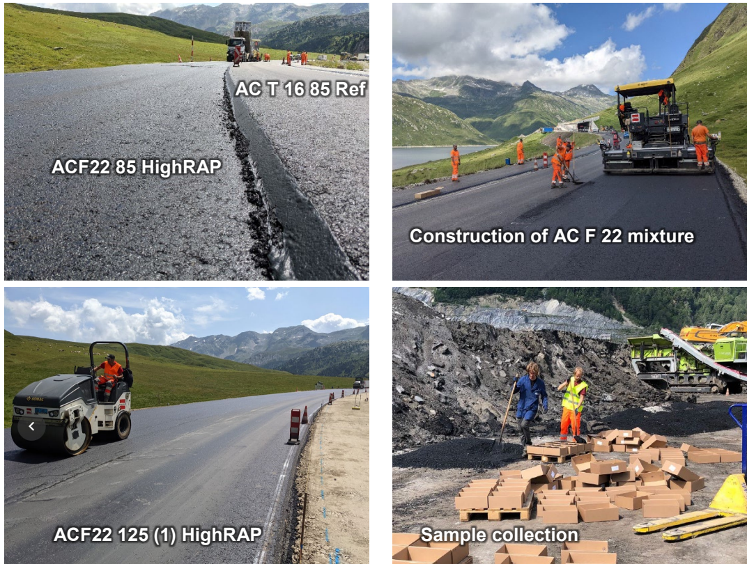
Fig. 150 Construction of Lukmanierpass test section
