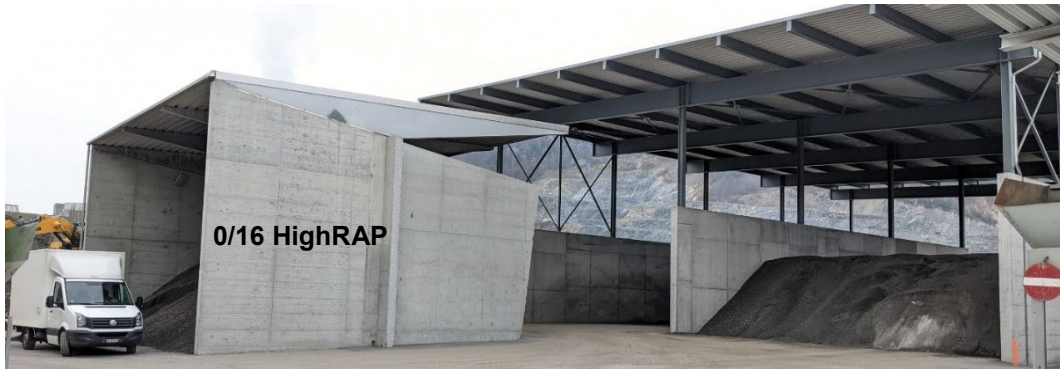
Fig. 145 Storage of the sampled reclaimed asphalt (0/16 HighRAP) for the Lukmanierpass test section in the Catram AG asphalt plant
