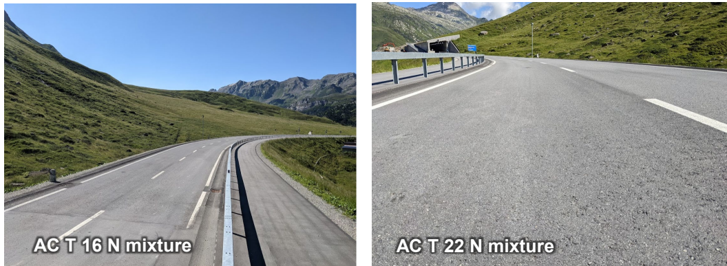
Fig. 151 Photos from inspection of the test site in July 2022 before the paving of wearing course
